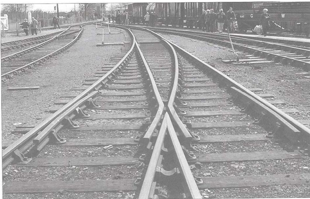
8. A more complicated set of points can be seen in the in the photograph below, which shows a double slip point where any track can be set to any other track. In this case the route set is for a train going away from the camera and taking the track to the left. Again, such points are used primarily in sidings and other slow speed areas where they save space, such points would not be seen on high speed main lines. One of the levers used to change the points can be seen on the right.
