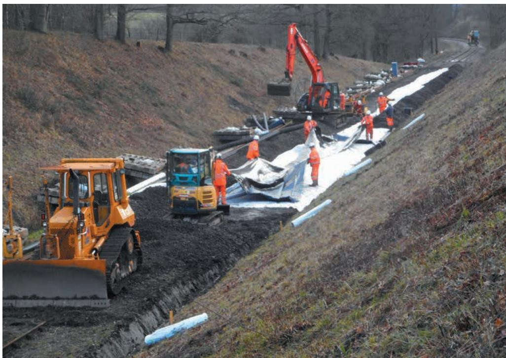
Looking north, showing the first cross drain being laid in at the south end of the cutting.
