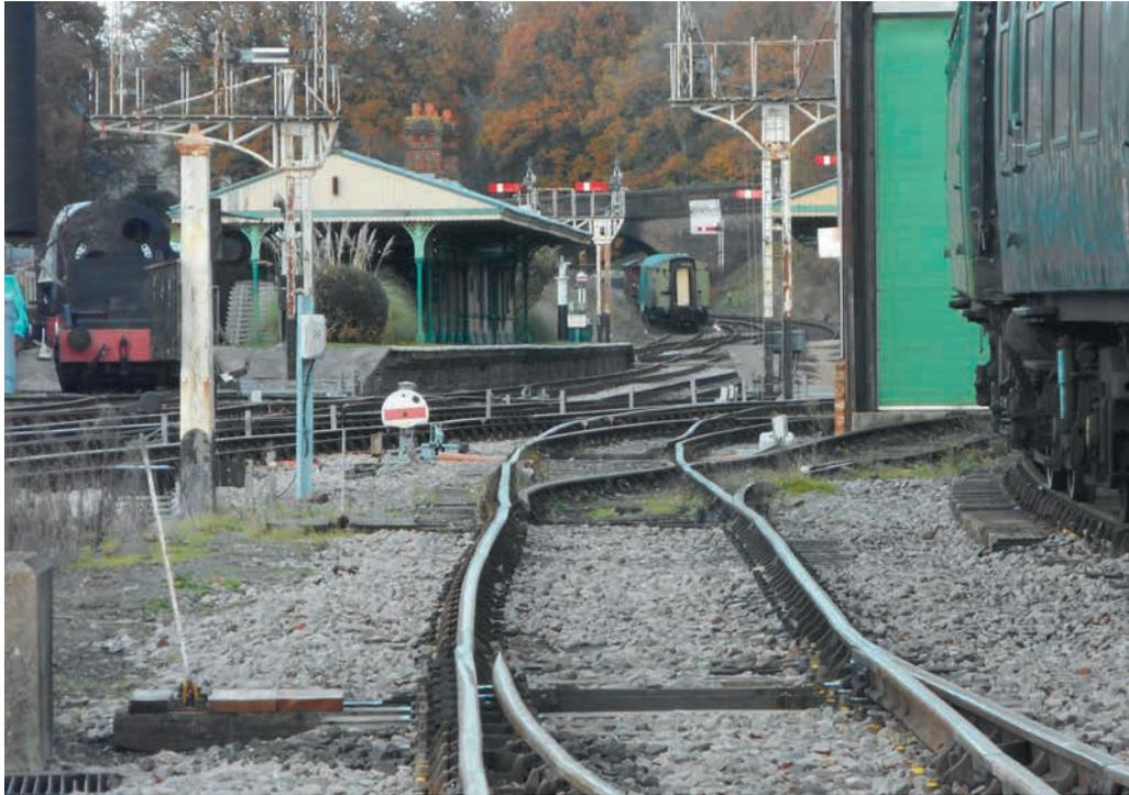
Due for renewal, the poor running in road from the station to the yard, with its visible 'kink'.
