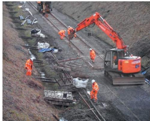
**ABOVE:** After bulldozing the ballast flat and compacting it smooth with the triple Wacker, the yellow line was painted on the ballast in line with the sleeper ends to help the team to place the sleepers accurately, as seen being craned in four at a time suspended from a lifting bar.
