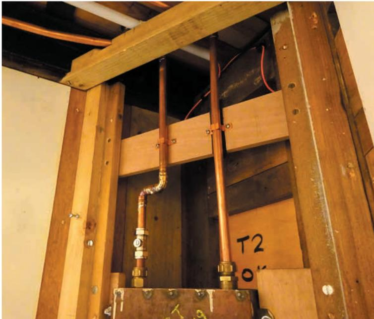
The cistern has been plumbed in to the newly-installed water tank in the ceiling above No 3687's lavatory. ALEX MORLEY
