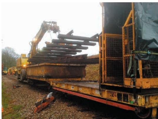
ABOVE: A half-panel is craned out to be transported off site and dismantled at a later date.
