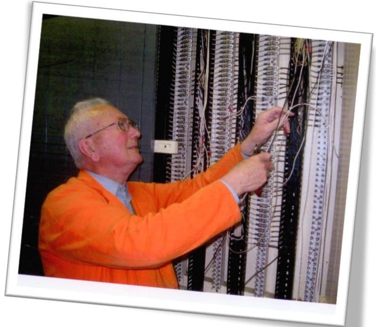
*Removing some temporary switch panel wiring underneath Horsted Keynes Signal Box in 2011, following the comprehensive overhaul of the lever frame*
