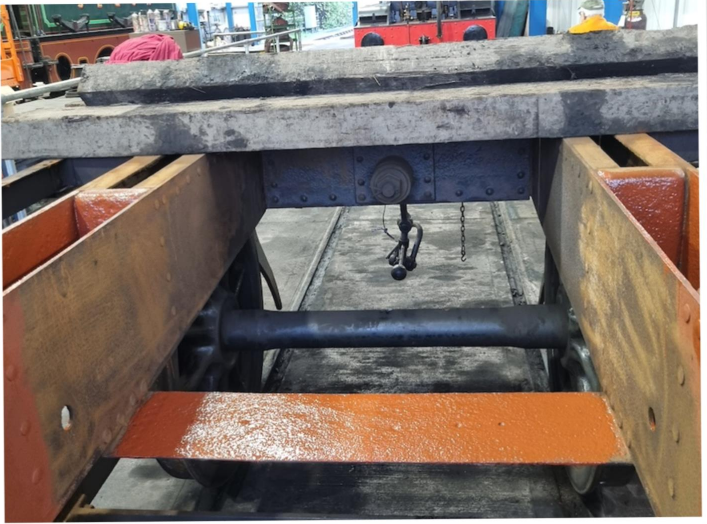
Above: Progress with cleaning and painting 541's inner tender frames. Photo: Steve Pilcher
