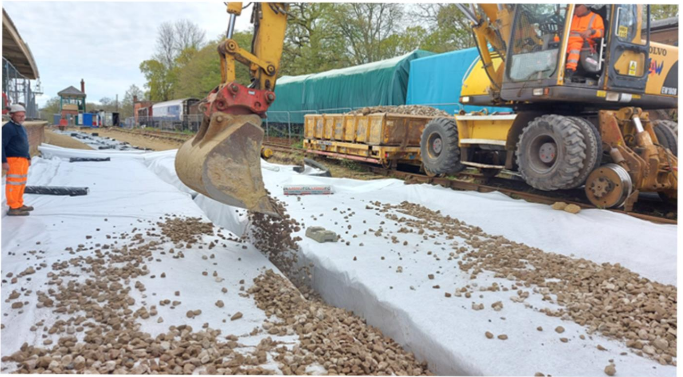
Above: The French drain being filled with track ballast on top of the waterproof membrane. Photo: Jon Goff
