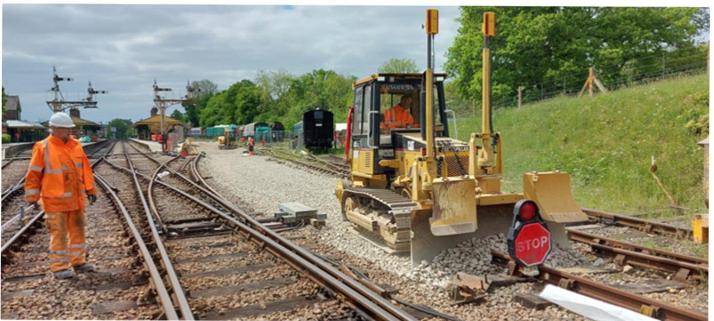
Above: The laser dozer at top end of the job with the stop board sitting on the end of the points. Photo: Jon Goff
